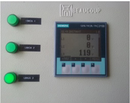
Figure 17 – Reading of electrical variables with power cut off
